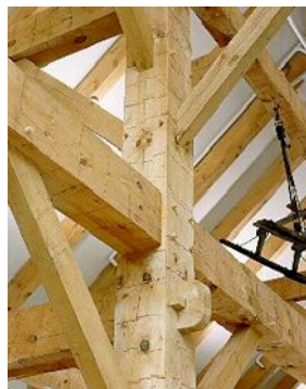
woodworking joints
